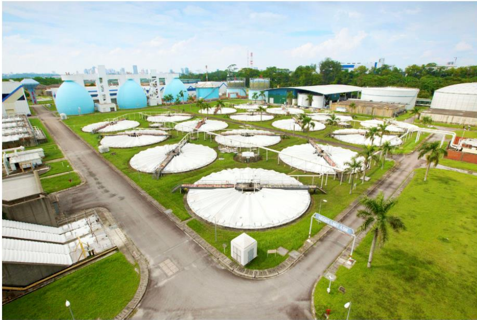
Existing Kranji Water Reclamation Plant and co-located NEWater Factory
